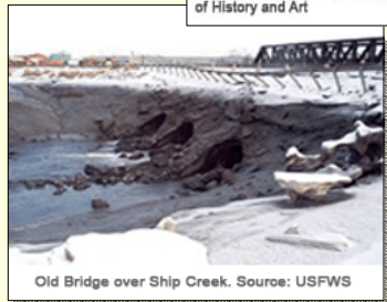
Old Bridge over Ship Creek. Source: USFWS
