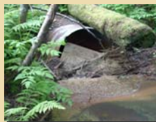
Fig. 5 (Above) A Culvert blocked with debris.
